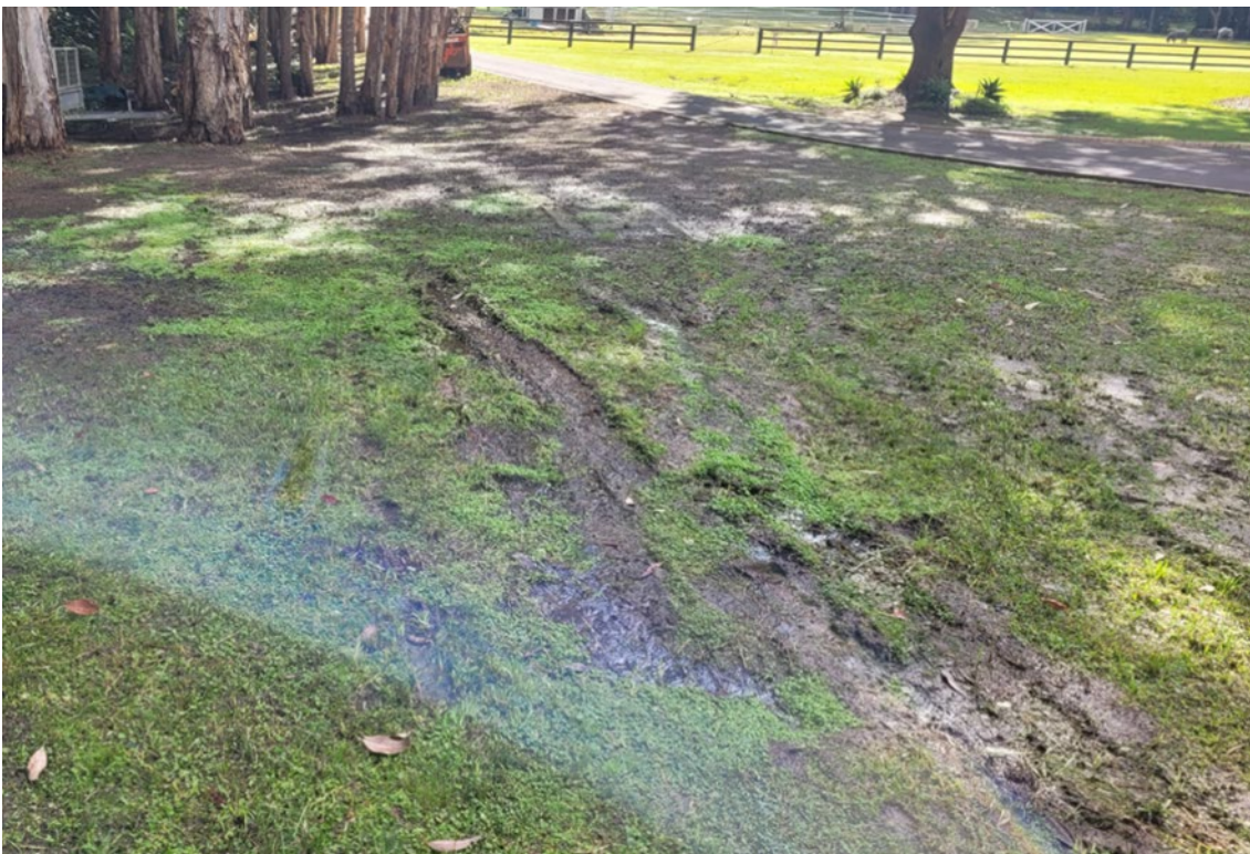
Figure A6–14. Damage to an absorption EAA system
