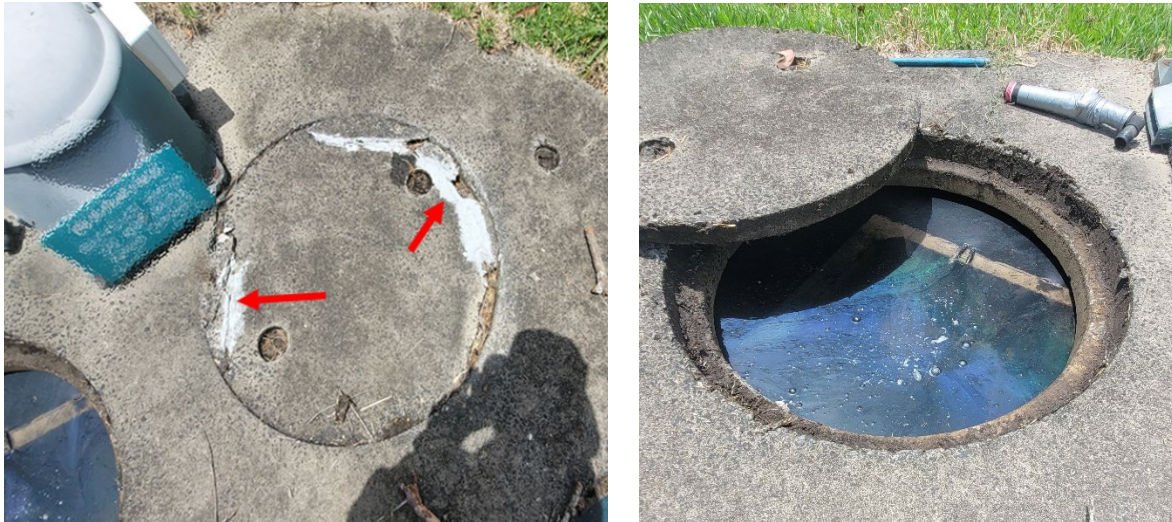
Figure A6–10. A damaged tank lid
