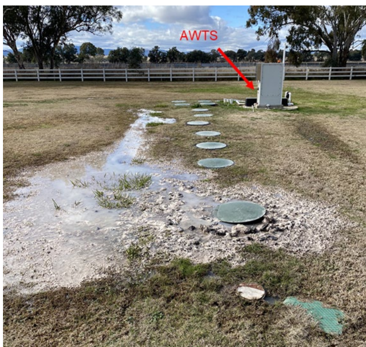
Figure A6-12. Sewerage leakage
