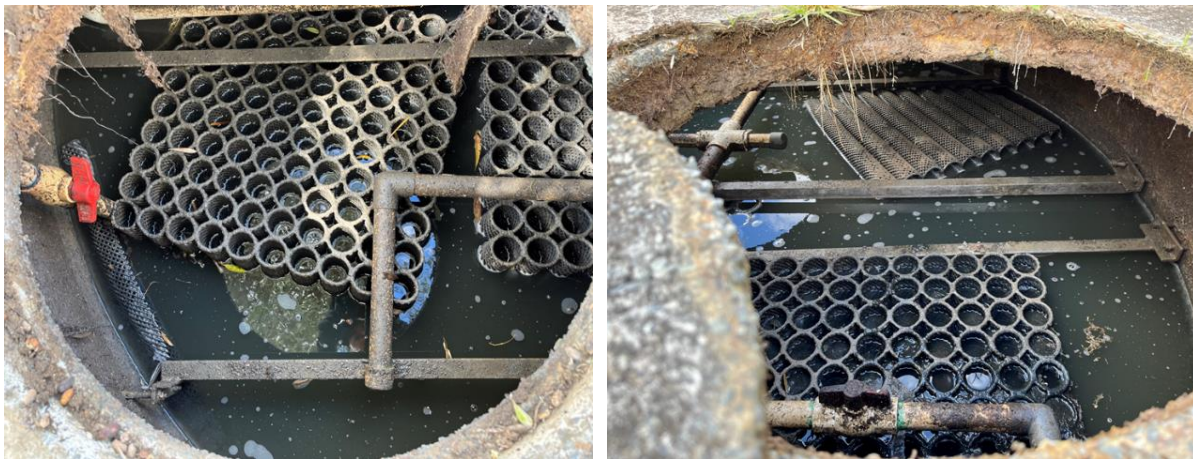
Figure A6-13. A secondary treatment system that has not been serviced properly
