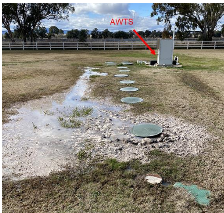
Figure A6-12. Sewerage leakage
