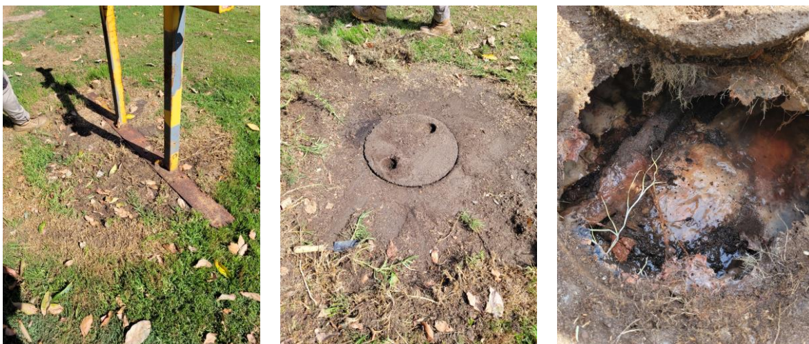
Figure A6-11. Tank issues caused by poor maintenance
