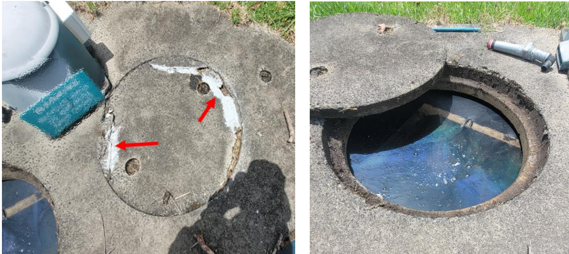
Figure A6-10. A damaged tank lid
